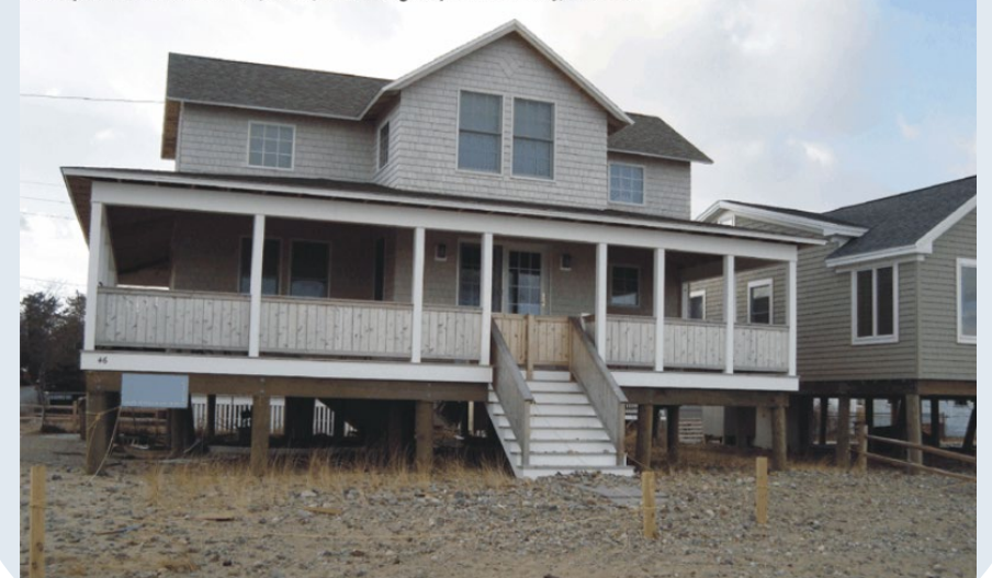
Example of Pile Foundation, Saco, ME. Image by P.A. Slovinsky, 12/2009.
